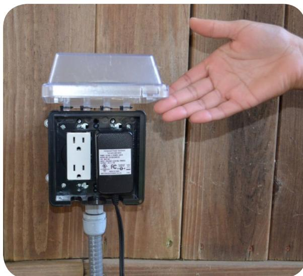
3. **Find Skirting Location For Control Panel:** Find a convenient location on the skirting just below the fiberglass lip of the spa. It is important that the location is near the access panel to the spa compartment allowing the cell cable to be routed appropriately. Rout the Cell Cable from the control panel through the spas access panel. Most access panels have a small gap at the bottom of the panel. See Picture Below.
